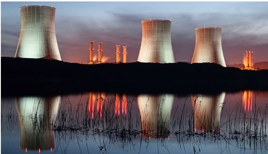
Image 3. Thermoelectric power plants require tremendous quantities of water to produce electricity.
