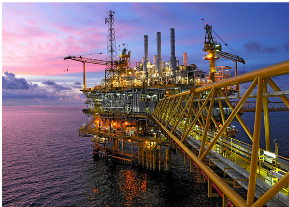
Space and weight are critical concerns topside. Moving flow-assurance operations off of the platform creates significant savings.
