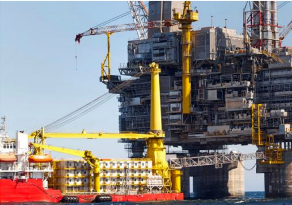
Flow-assurance chemicals are typically fed from supply tanks on FPSOs and are metered via surface-dedicated chemical injection pumps. (Images courtesy of IDEX Corporation)
