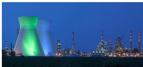
2. Most power plants are located near an abundant water source, such as a river, lake or stream.
