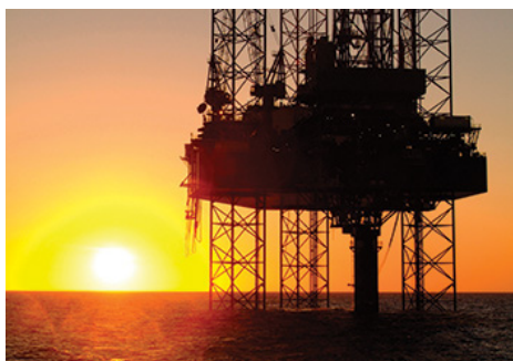
As oil & gas producers look to triple their production, offshore end users will need more powerful pumps. (Article images courtesy of Milton Roy.)
